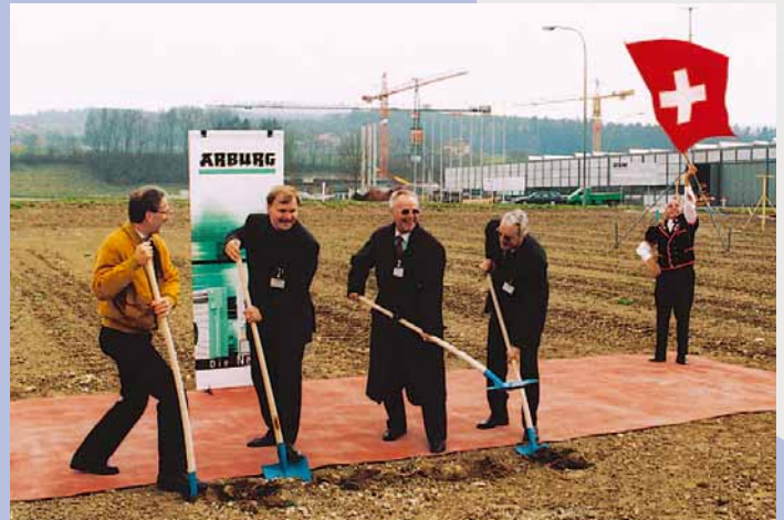
Digging with great gusto – Eugen Hehl (2 nd from right), branch manager, Peter Moser, (right), ARBURG's senior project manager, Manfred Wolfer (2 nd from left) and the architect in charge, Jörg Jost (left) boldly took hold of their shovels on the building site in the Swiss town of Münsingen.
