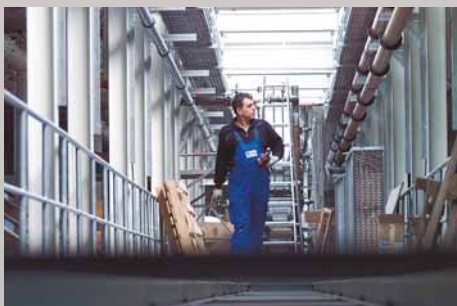
The finishing touch – tradesmen know exactly where it's needed. And everyone does their bit to ensure that the work is completed quickly
